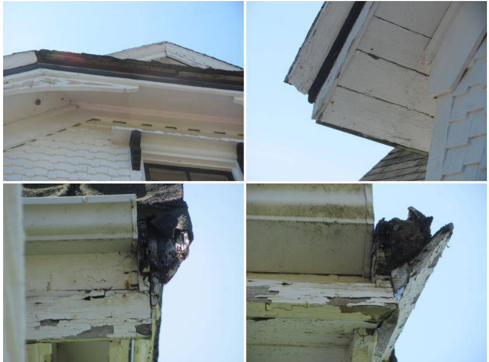
Wood materials. Damage noted, Loose or deteriorated material is noted at the trims of the building. Moisture stains/damage noted under eaves, Paint/finish is needed.
