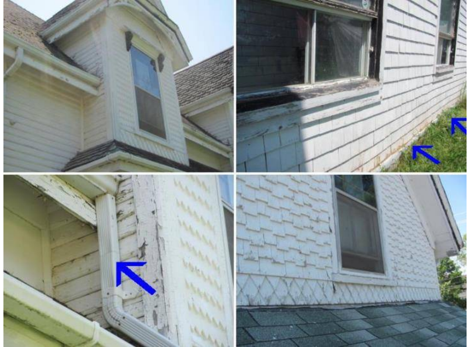
Damaged areas of siding are seen.
